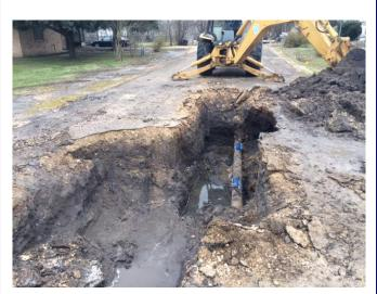
City Crew fix a 6" main water line on Colfax Street. The line was fixed "Hot" meaning under high pressure.
